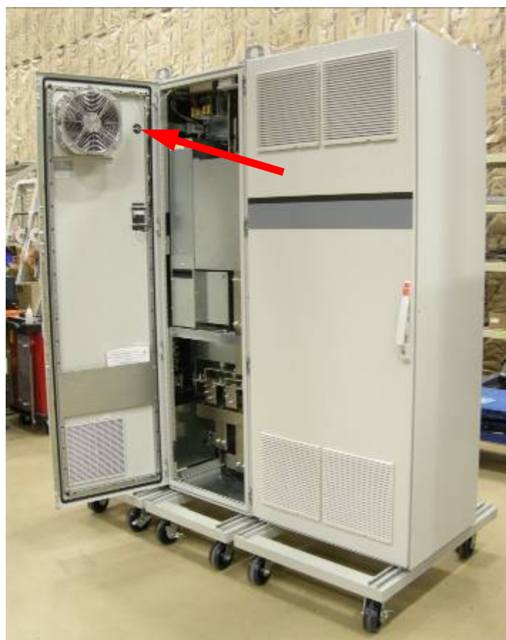
Figure 1. Location of USB feed-through hole.
