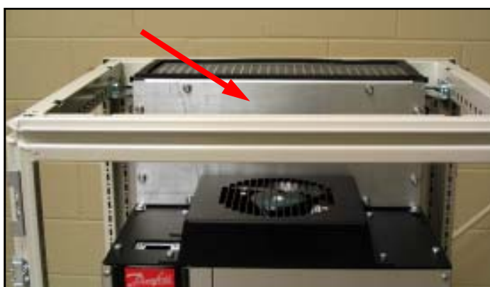
Figure 21. Top duct closing plate installed
