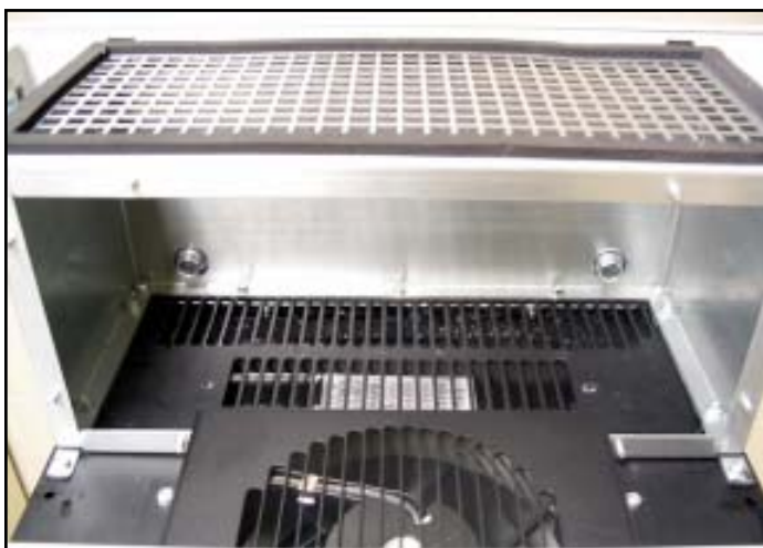
Figure 18. Top duct installed
