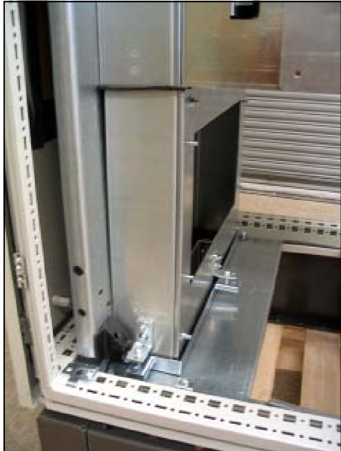
Figure 26. Duct work temporarily installed to mark cut-out on the gland plate
