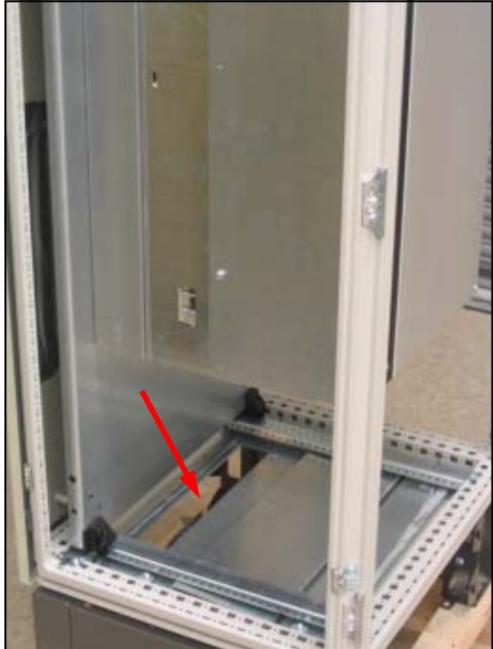
Figure 27. Enclosure bottom cutout
