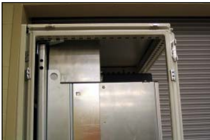
Figure 13. Top duct work and enclosure top installed
