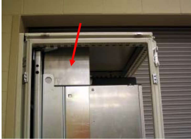
Photo 8. Top duct work and enclosure top installed.
