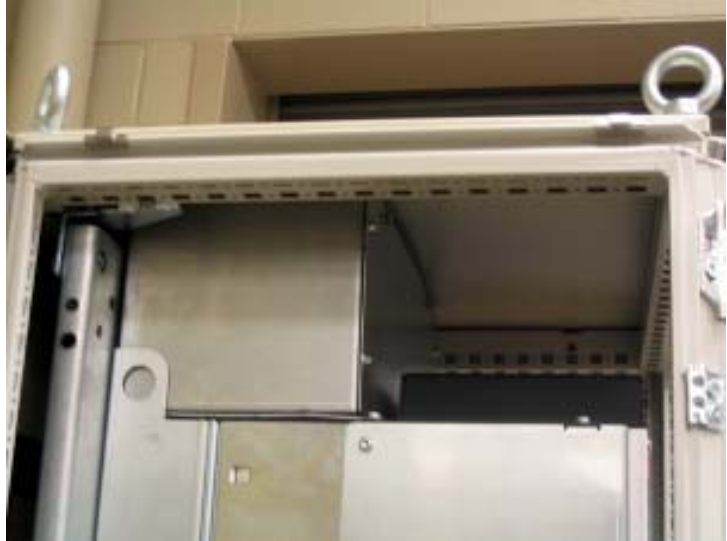
Photo 18. Enclosure top installed.
