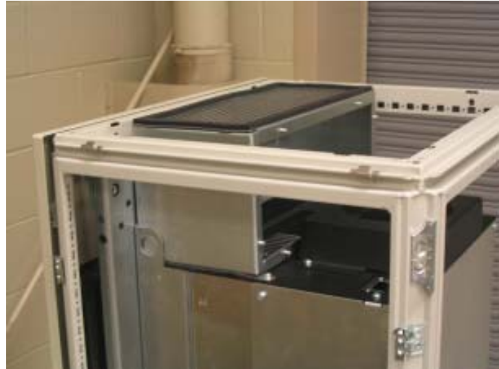
Photo 15. Top duct installed.
