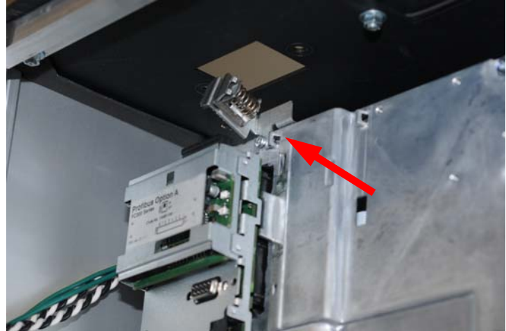
Photo 6. Installed shield termination/strain relief.
