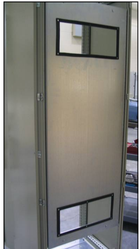
Figure 10. Back of drive mounting plate with gaskets installed
