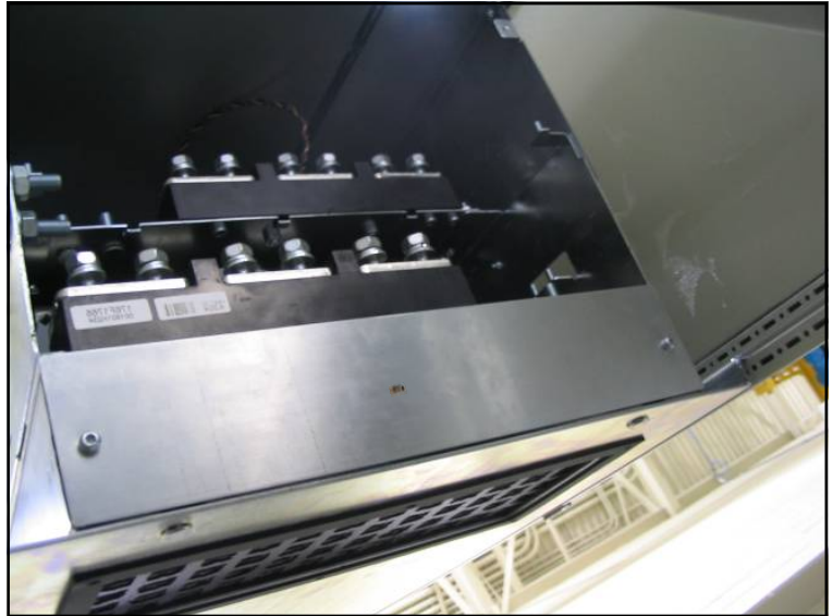
Figure 16. Bottom air inlet cover installed
