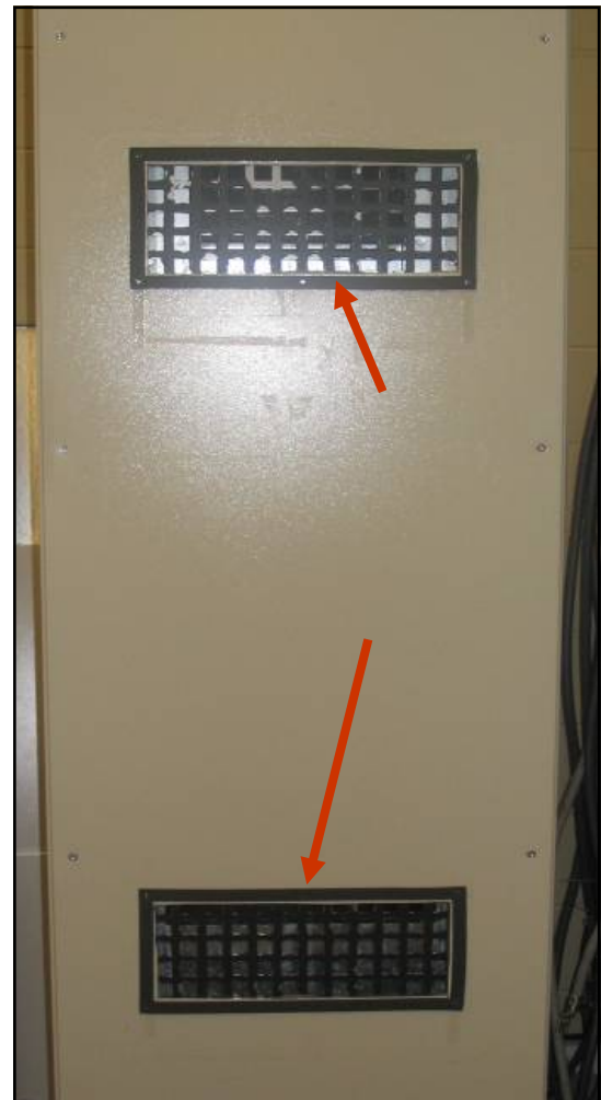
Figure 18. Gasket installed on the outside of the rear panel
