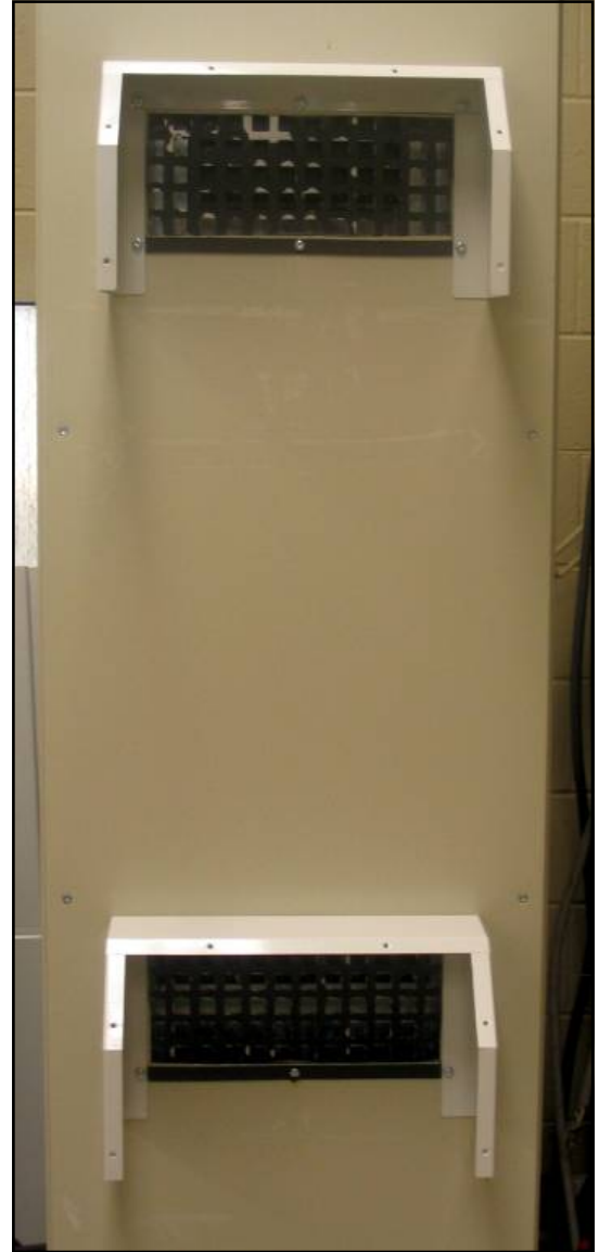
Figure 19. Deflector frames installed on top and bottom openings
