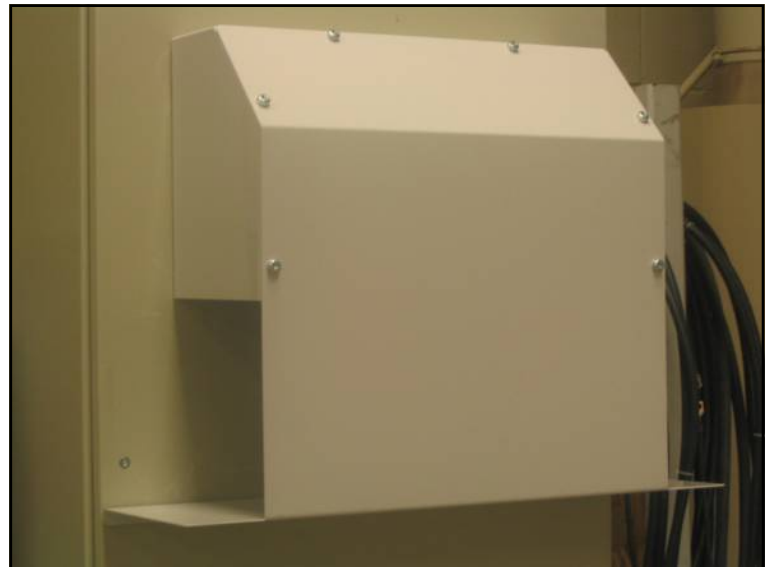
Figure 21. Upper deflector assembly installed
