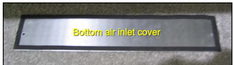
Figure 3. Bottom air inlet cover (with gasket)
