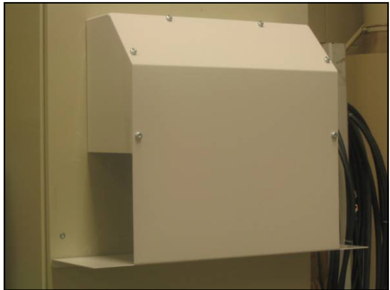
Figure 19. Upper deflector assembly installed
