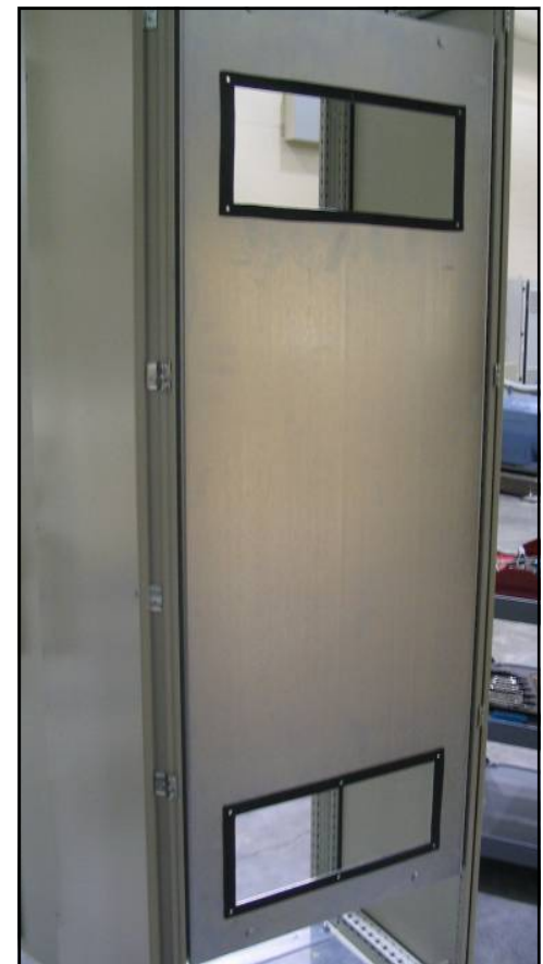
Figure 8. Back of drive mounting plate with gasket installed
