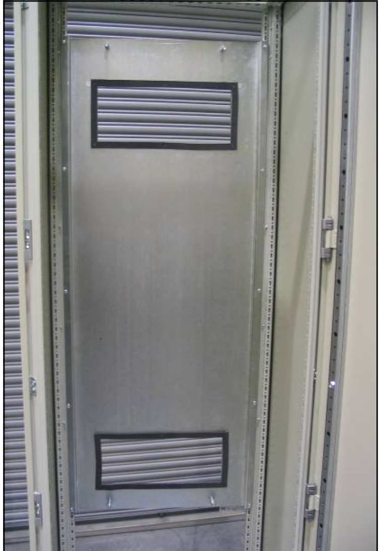
Figure 6. Drive mounting plate installed with rear panel of enclosure removed
