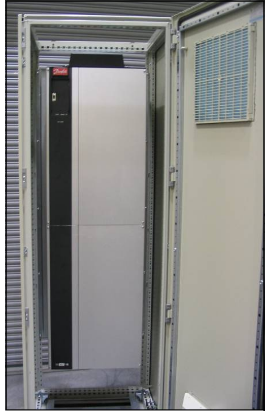
Figure 9. Drive installed on mounting plate
