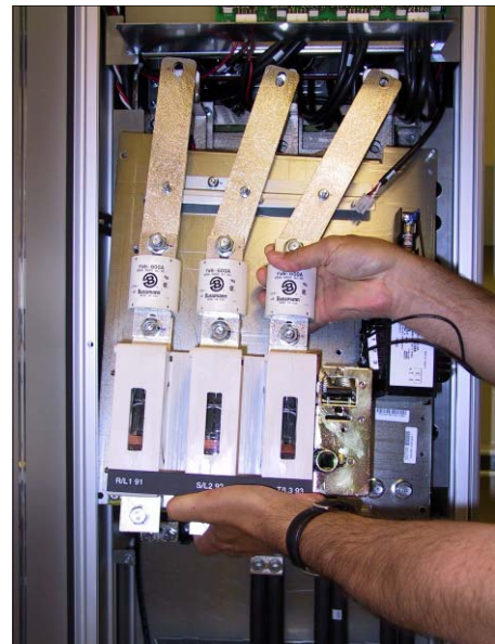
Photo 8. Installing of kit containing Disconnect and Fuses
