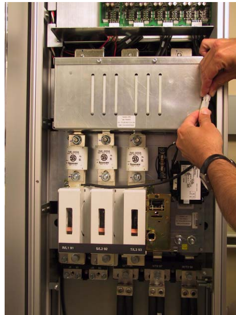
Photo 11. Reconnecting Fan Transformer Wiring
