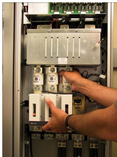
Photo 10. Installing Input Plate with Disconnect, Fuses and RFI
