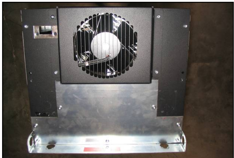
Figure 3. Top cover plate installed
