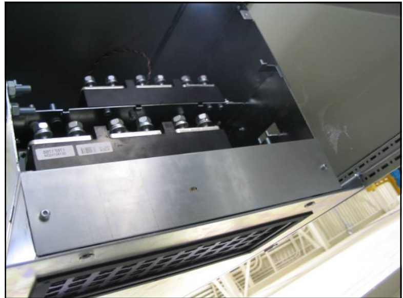
Figure 12. Bottom air inlet cover installed
