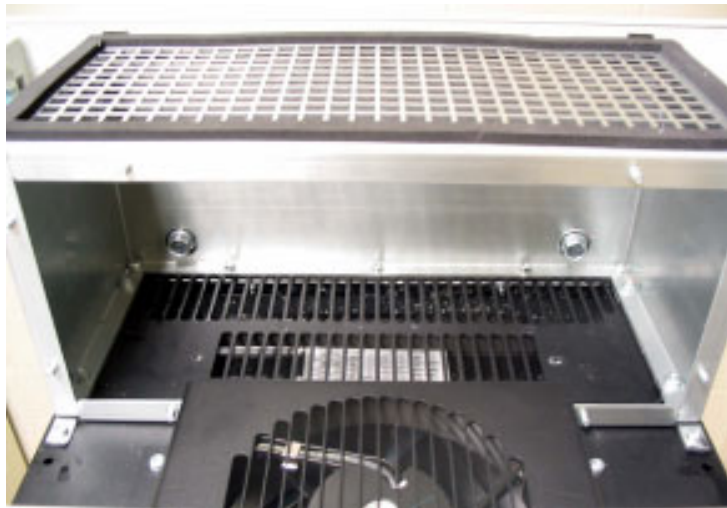
Photo 14. Top duct installed.
