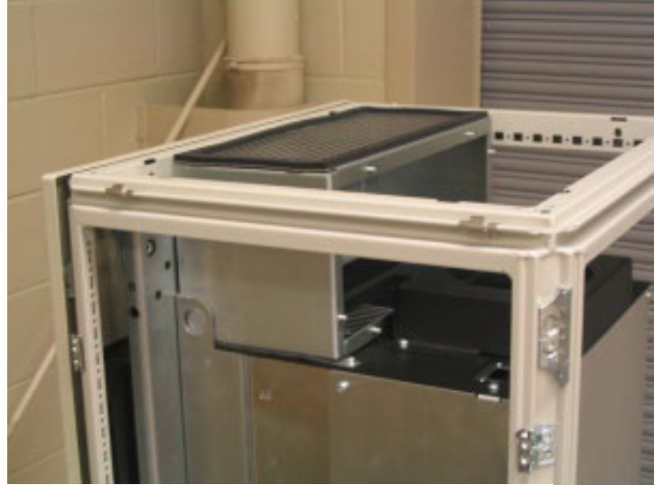
Photo 15. Top duct installed.
