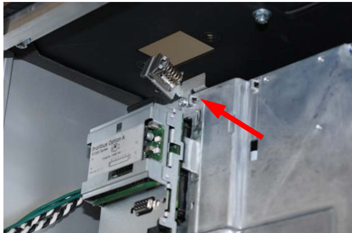
Photo 6. Installed shield termination/strain relief.
