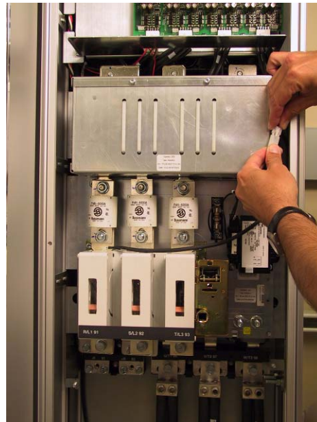
Photo 11. Reconnecting Fan Transformer Wiring
