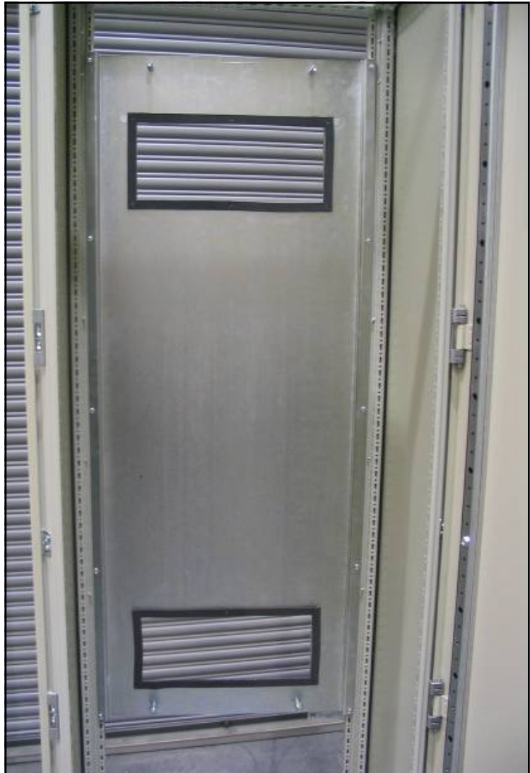
Figure 6. Drive mounting plate installed with rear panel of enclosure removed
