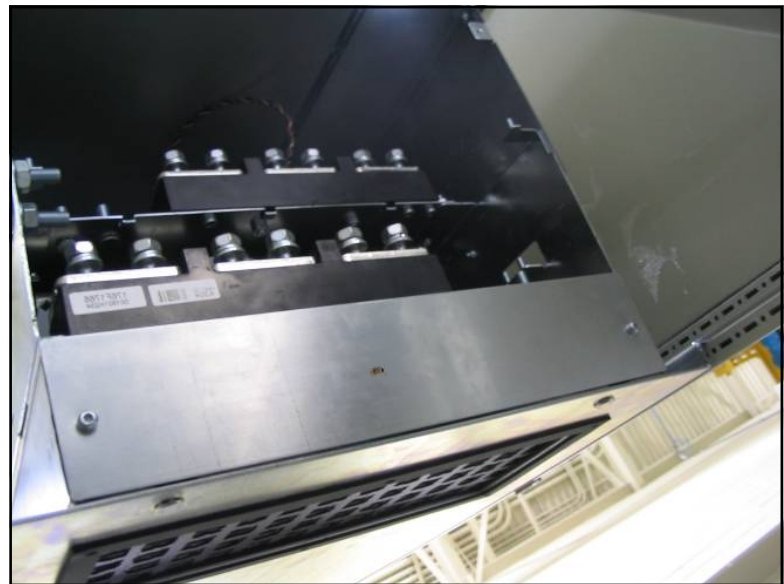
Figure 16. Bottom air inlet cover installed
