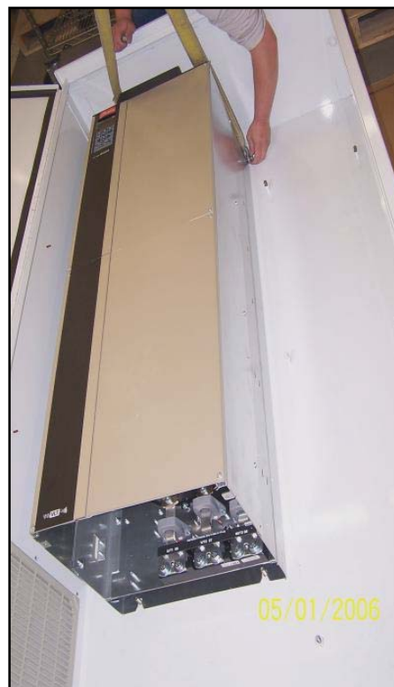
Figure 9. Drive installed in enclosure
