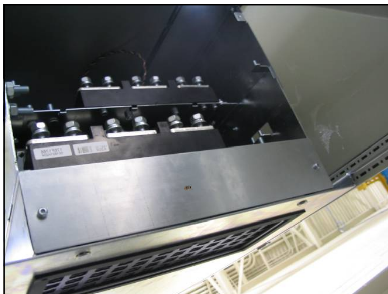
Figure 12. Bottom air inlet cover installed
