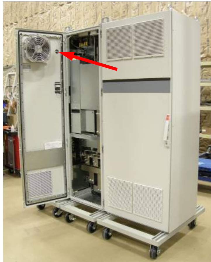
Figure 1. Location of USB feed-through hole.
